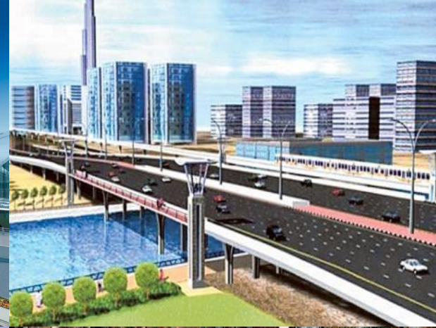
Dubai Creek Bridge- Business Bay
